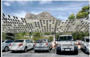
Photo Voltaic Covered Parking
